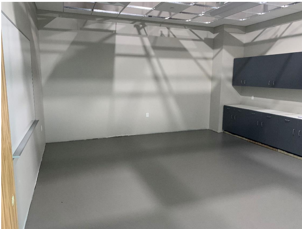
28. Area 5 – Casework, marker board, and resilient flooring appear to be installed in second floor staff work room.
