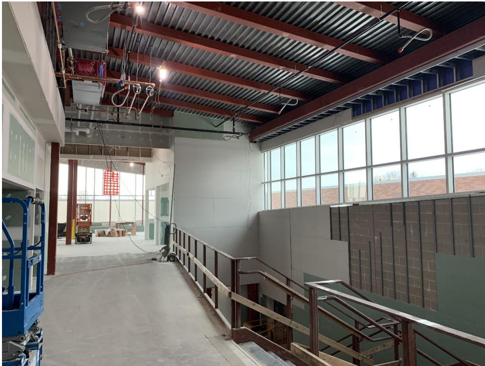
50. Area 1A – Taping and mudding in LMC in progress. Perimeter seat wall in progress.
