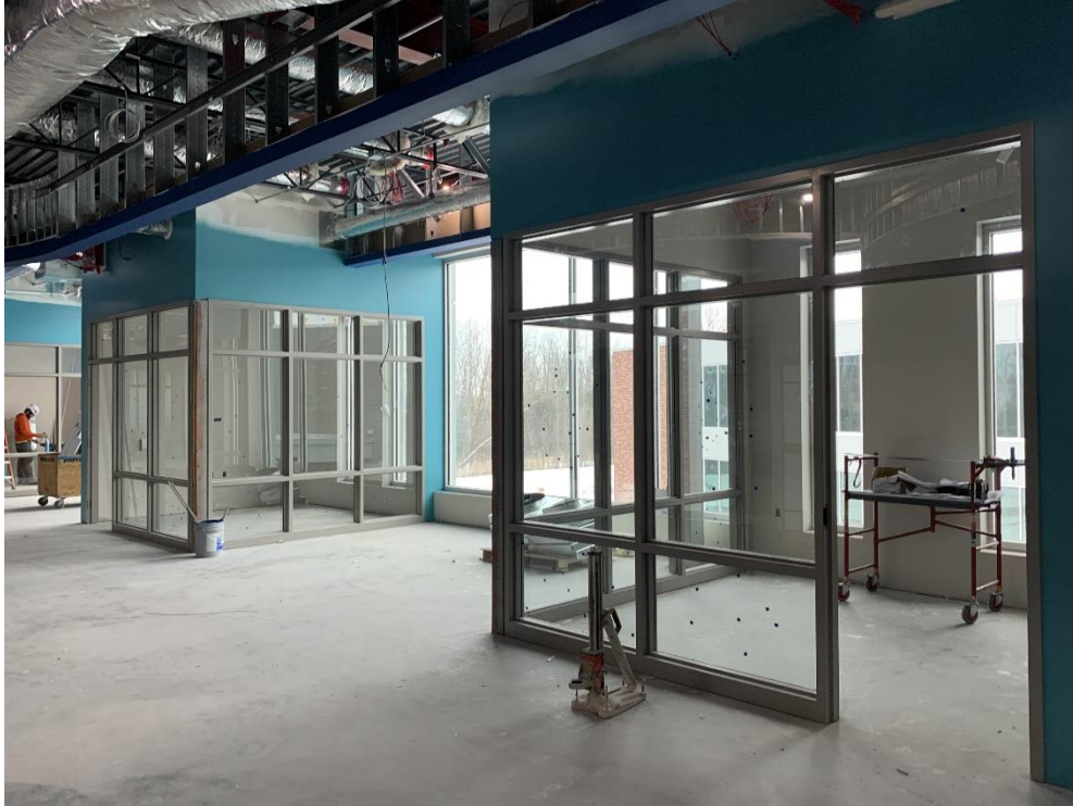
36. Area 4 – Casework and sliding door system install in second floor classrooms in progress.
