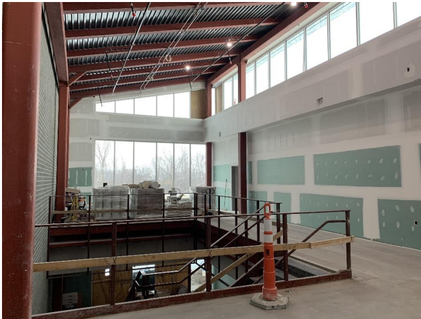
48. Area 1B – Gyp board taping and mudding in second floor center spine in progress.
