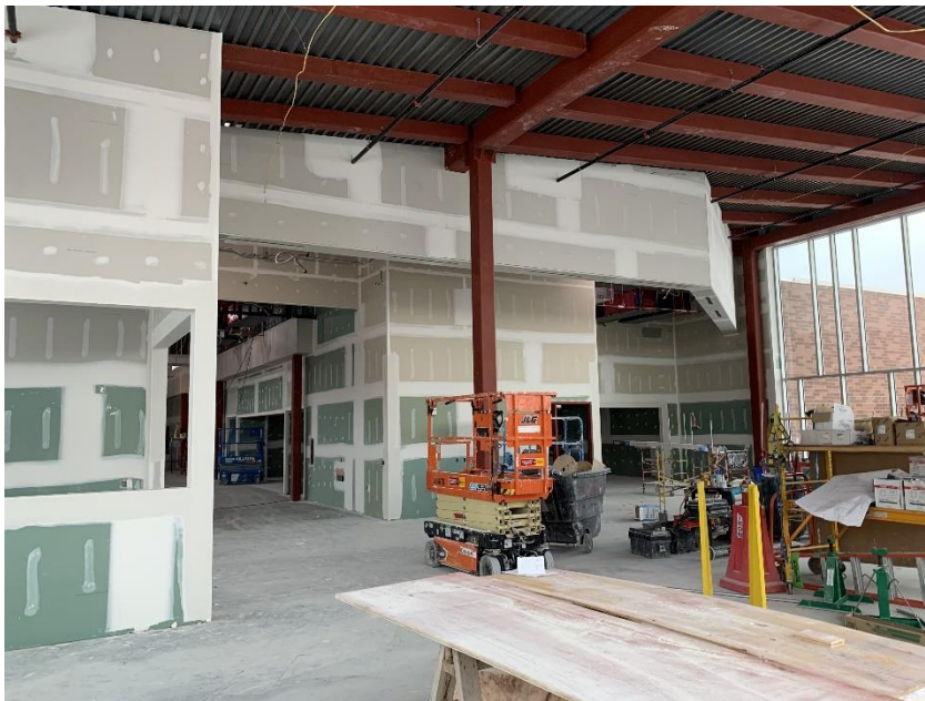
50. Area 1A – Taping and mudding in LMC in progress. Perimeter seat wall in progress.
