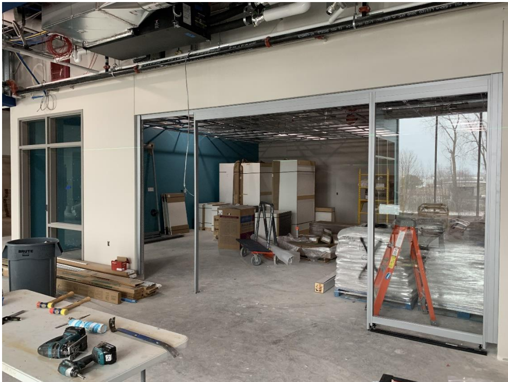
36. Area 4 – Casework and sliding door system install in second floor classrooms in progress.
